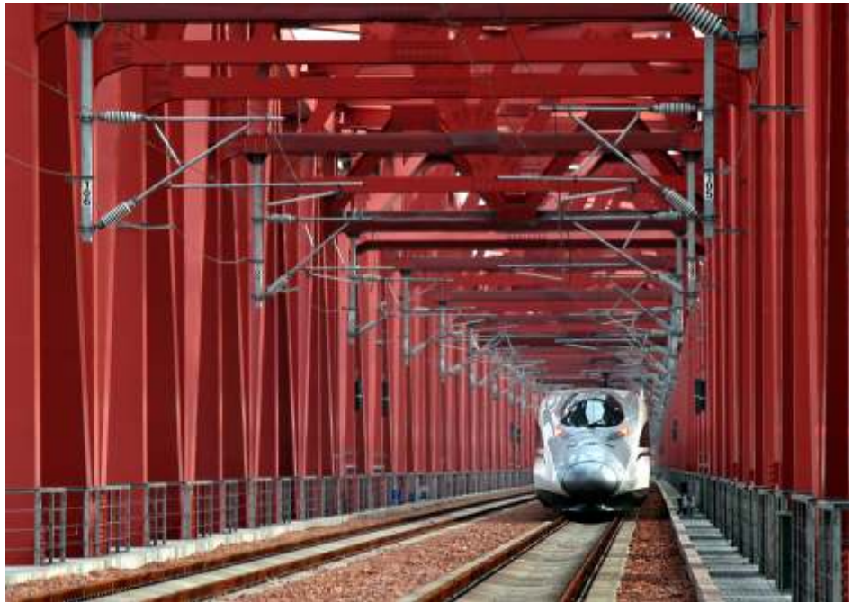
A CRH train runs on a bridge on the Yellow River of the Zhengzhou-Jiaozuo railway line, central China's Henan Province, May 4, 2015.
